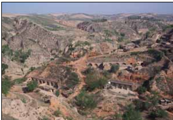
The traditional cave dwellings in the village of Dang Jia Shan. Photo courtesy of Anrong Dang.
